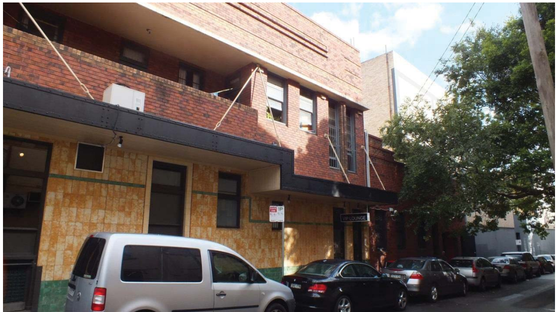
Figure 20 — the north-western elevation, sees from Dunblane Street. NBRSPARTNERS April 2014
