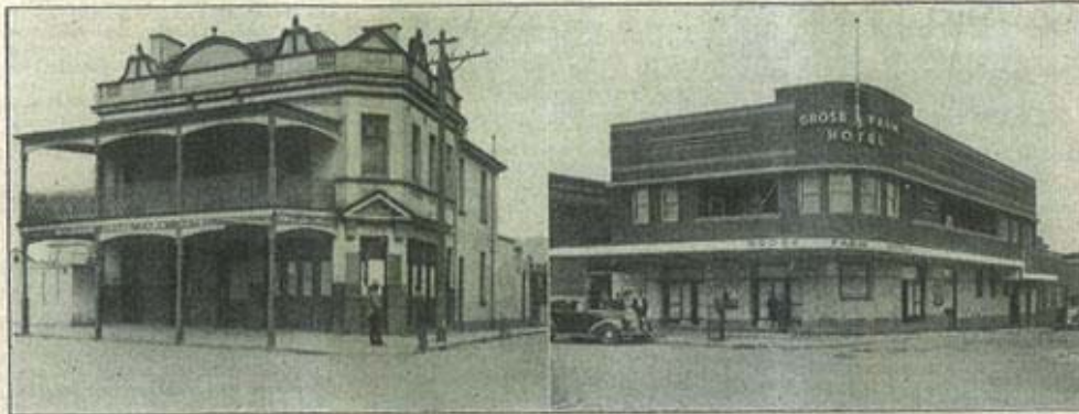
THE STORY of hotel improvement is best told by the pictures. On the left is the old Grose Farm Hotel, which is to be demolished, and the picture on the right is the new Grose Farm Hotel, opened for business on November 6. It is on a new site further along Missenden Road, Camperdown.
