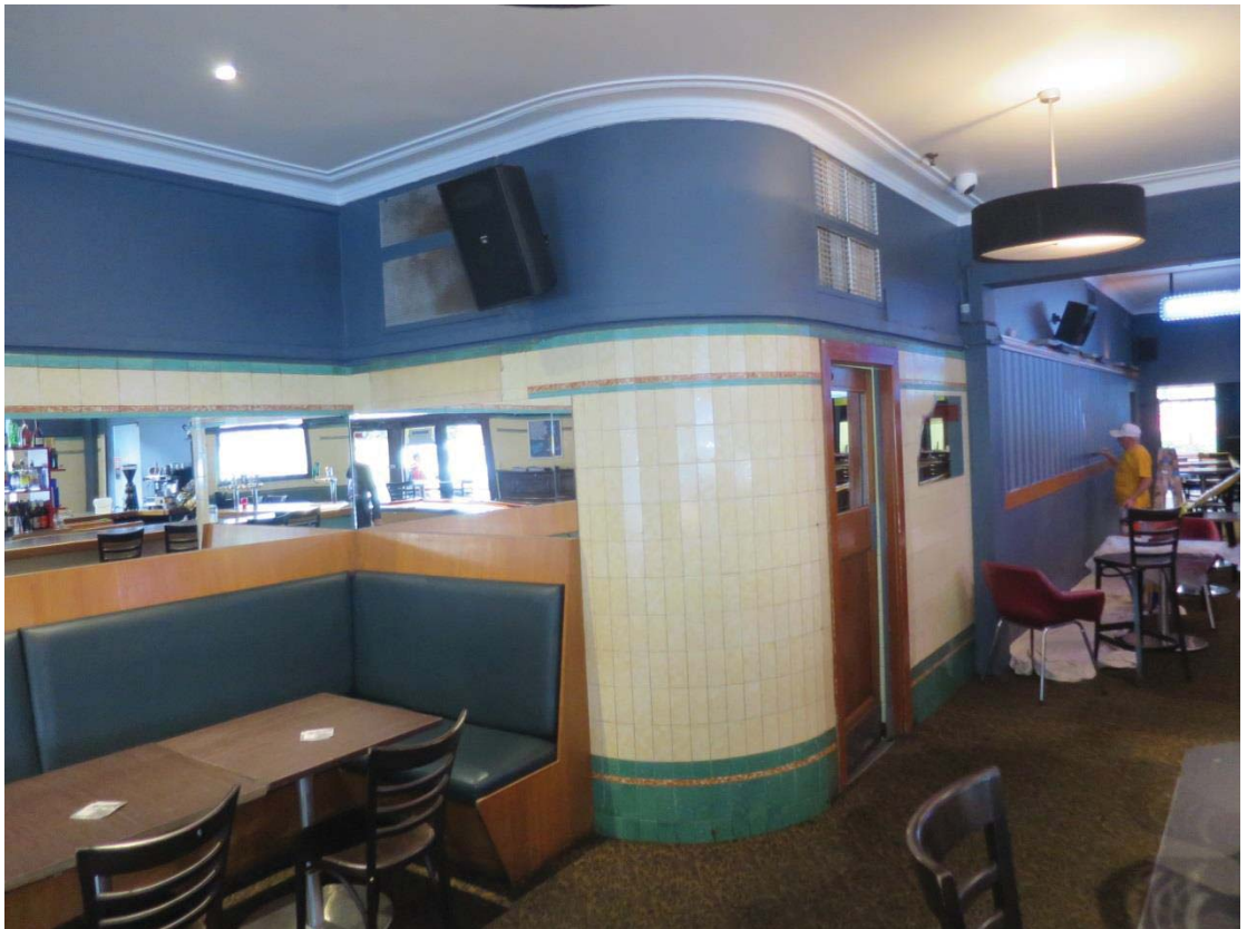
Figure 9 — the southern wall of the bar, featuring original wall tiles, timber door and cornice. Other fixtures in this view have no heritage significance.
