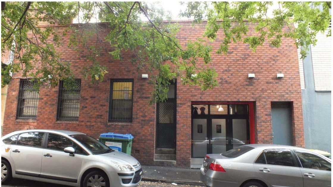
Figure 5 — north-west elevation of the single-storey section that is the site of the proposed serviced apartment development. The opening for the original garage has been re-glazed as a bar entry. NBRSPARTNERS April 2014
